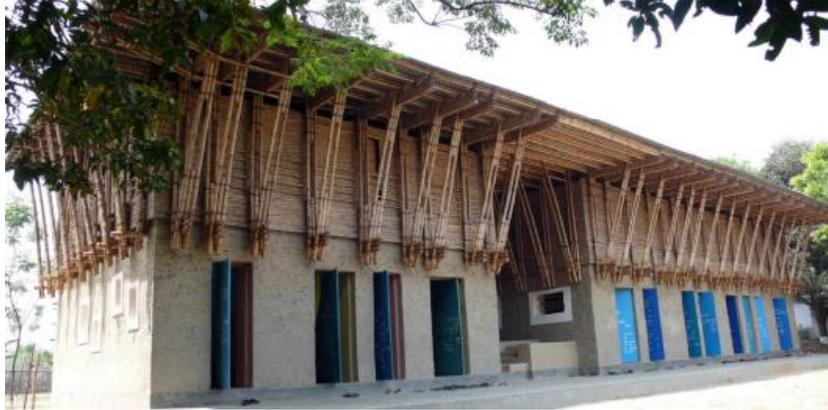
The building began with a small masonry foundation which was built on using a mixture of straw and dirt. This was left to harden for a week allowing the lower base to become strong. A ceiling for the ground floor was made with a triple layer of bamboo canes.
